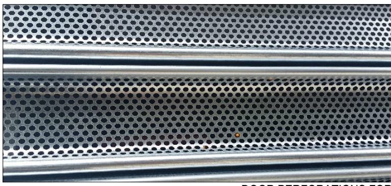
DOOR PERFORATIONS FOR VENTILATION REQUIREMENTS
