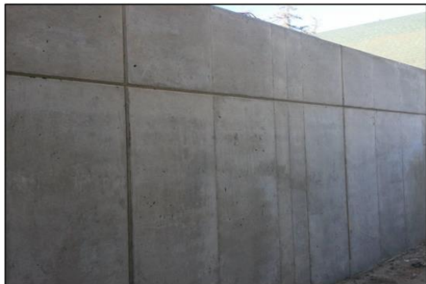
SMOOTH CONCRETE FINISH
