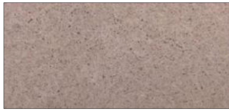
BOARD FORMED CONCRETE COLOR
